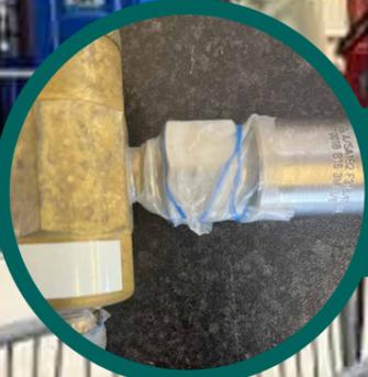
Leak detection tape around threaded joints
