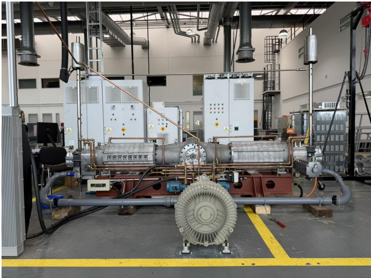
Figure 2. Installation at CEME
