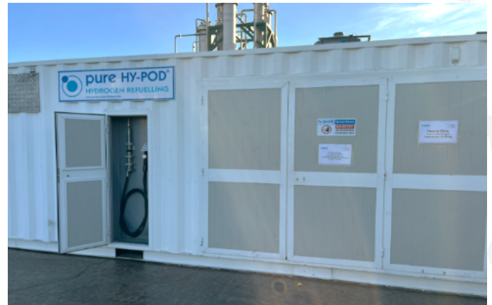
Figure 6 - Hydrogen Storage and Compression Processing Unit
