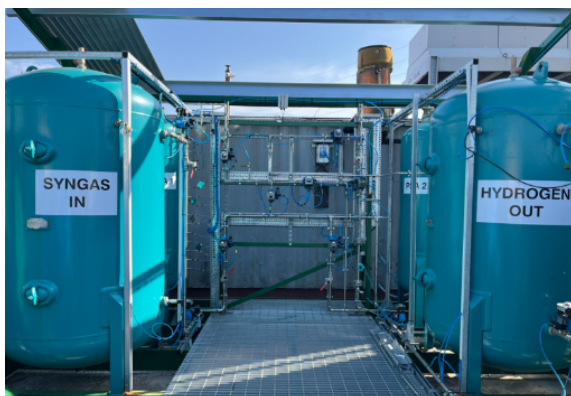
Figure 5 - Pressure Swing Adsorption Columns
