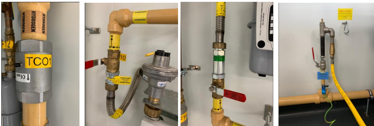
Figure 20 - Excess flow valves (2 nd from left onwards) and Thermal cut off valves (far left)
