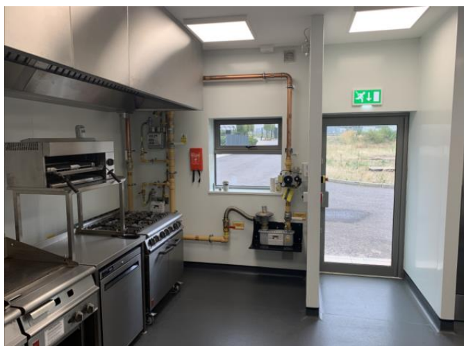
Figure 9 – View of the internal pipework, metering installation and associated equipment
