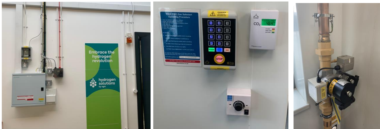
Figure 21 – Prove system (far right), control system (middle) and power system (left)
