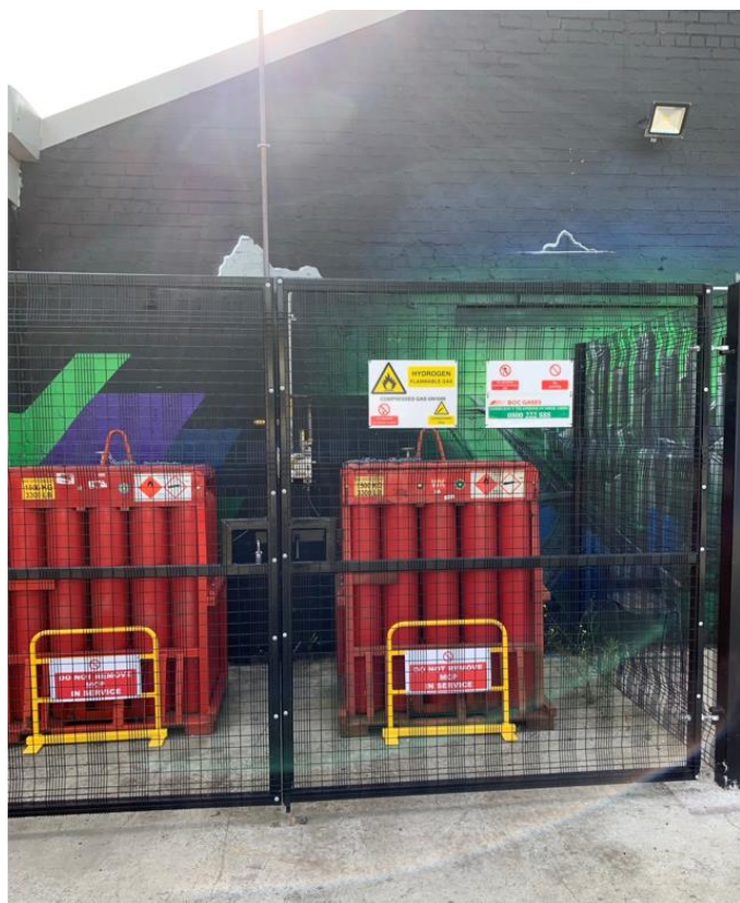
Figure 5 - Multi cylinder pallet (MCP) – 15 cylinders containing ~9kg of H 2 .
