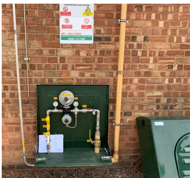
Figure 7 - 2 bar – 50 mbar boundary regulator.
