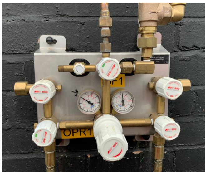
Figure 6 - MCP control panel – reduces the pressure from 175 bar to 2-3 bar.
